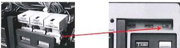
Figure 7 – Breakers with Shunt Trip or UVR in "third" far right accessory position
